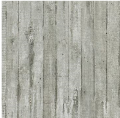
CONCRETE – VERTICAL BOARD FORM PATTERN
