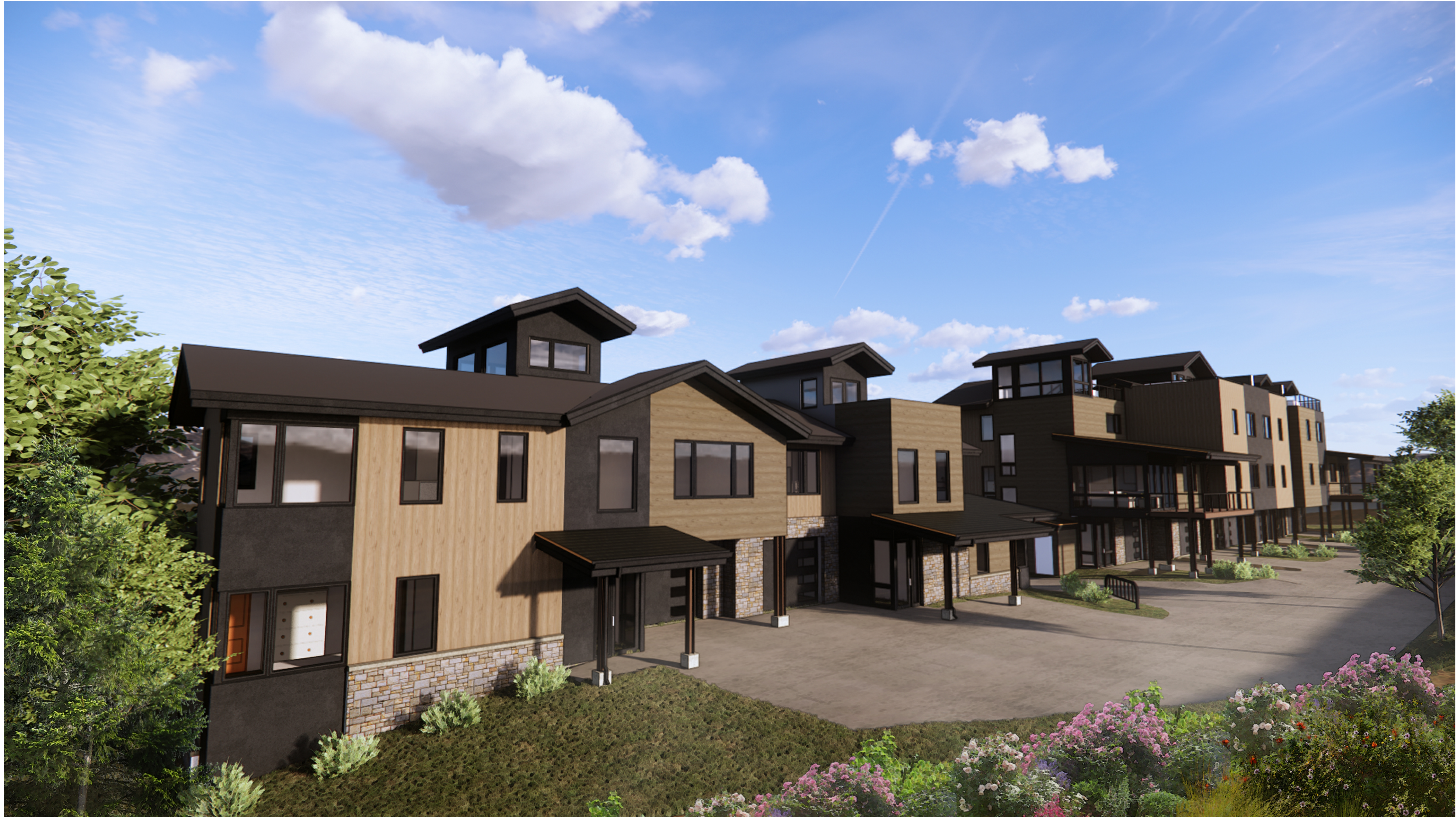
SOUTH BLDG LOOKING WEST
