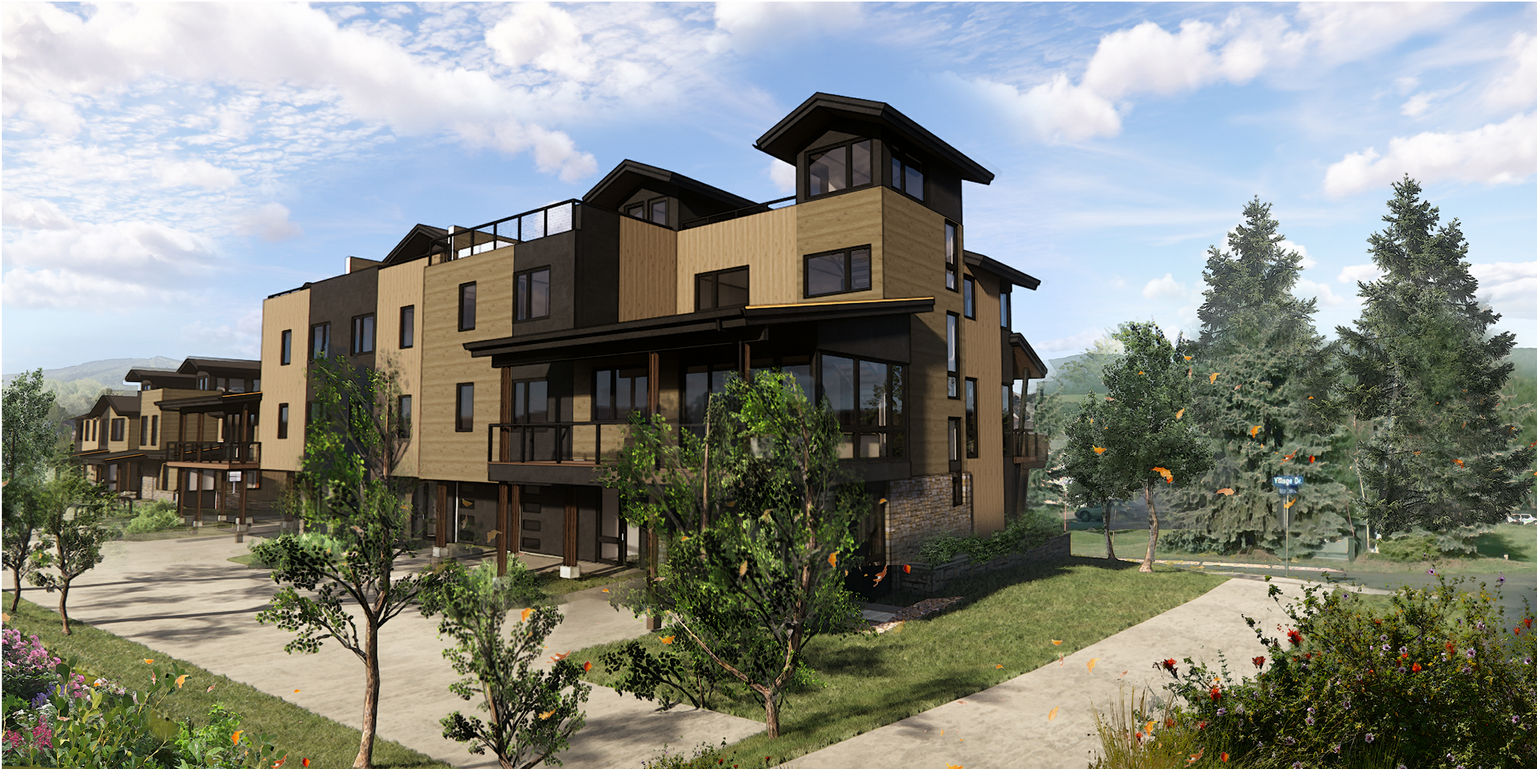
NORTH BLDG LOOKING WEST
