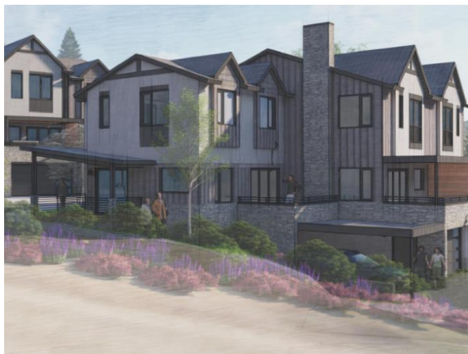
Building 2 – North Façade
