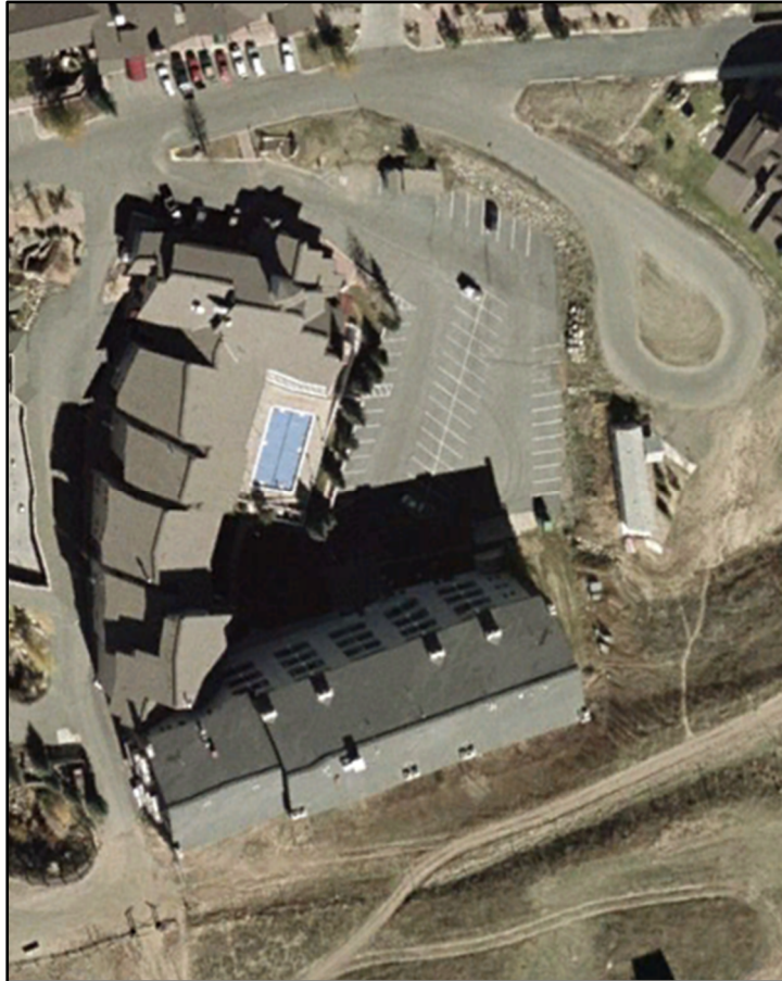
Figure 2: Thunderhead Lodge and Condominium prior to demolition.
