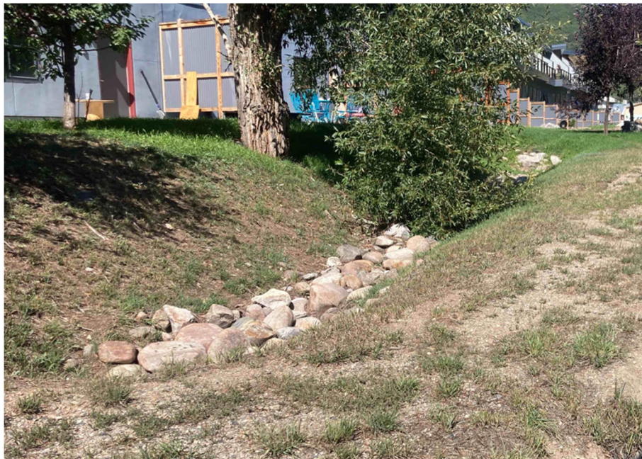
Existing Armored Swale Hand Remove Sediment
