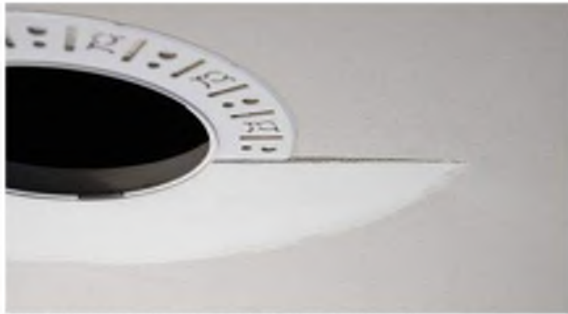
Partially finished mud ring, showing cross-section detail.
