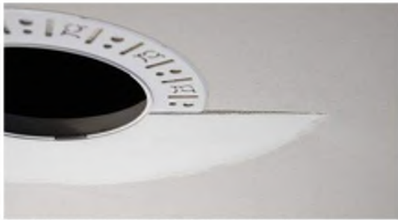
Partially finished mud ring, showing cross-section detail.
