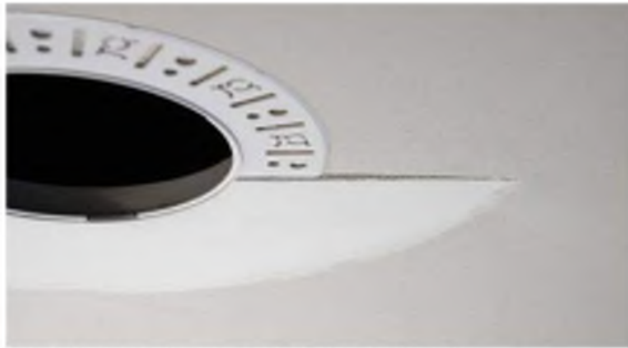
Partially finished mud ring, showing cross-section detail.
