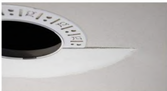
Partially finished mud ring, showing cross-section detail.
