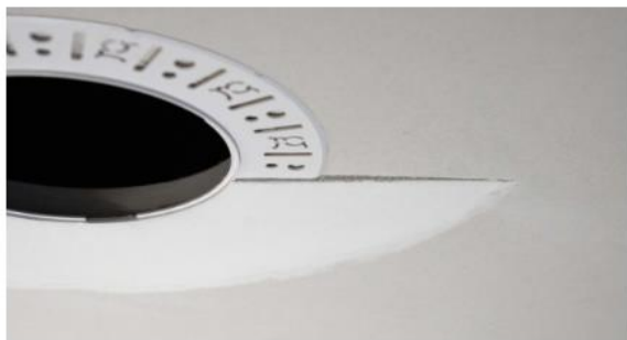
Partially finished mud ring, showing cross-section detail.
