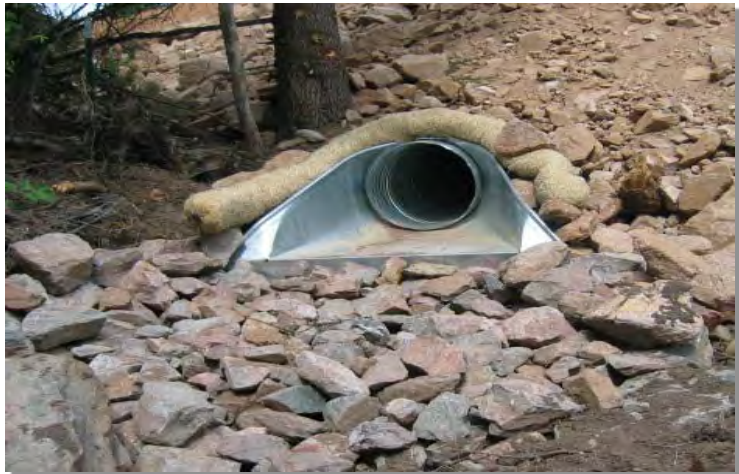
Photograph TOP-1. Riprap outlet protection.
