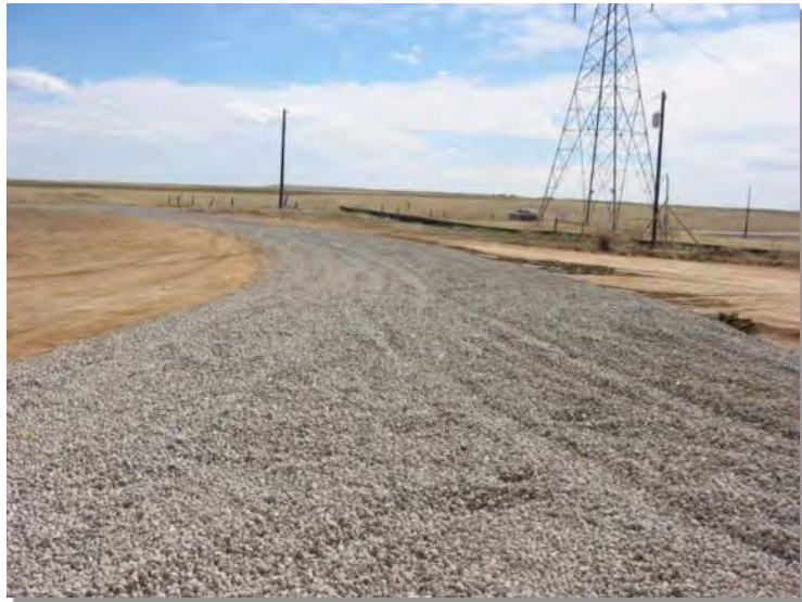
Photograph SCR-1. Stabilized construction roadway.
