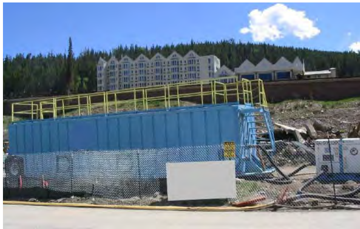
Photograph CT-1. Proprietary chemical treatment system being used on a construction site with sensitive receiving waters. Photo courtesy of WVE.
