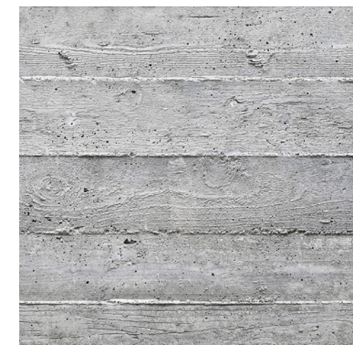
④.1 Concrete- Board Shuttered Concrete.
