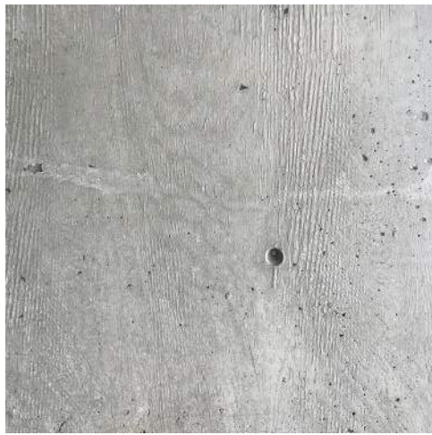
4.1 Concrete - All form work to be first use Tolko T-PLY Pro Oiled & Edge Sealed (OES) Premium DFP Plywood. Species and Grade Stamp: DFP CSA 0121, CCPTS
