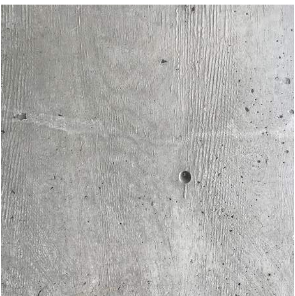
④ Concrete - All form work to be first use Tolko T-PLY Pro Oiled & Edge Sealed (OES) Premium DFP Plywood. Species and Grade Stamp: DFP CSA 0121, CCPTS
