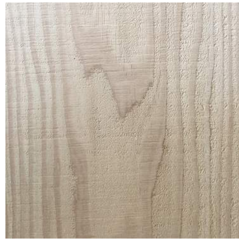
2.2 Roughsawn Solid DF - C Clear or better - Balcony Support and 2x6 Studs at Sauna Screen
